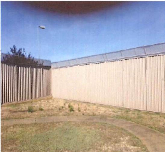
After Photograph showing 600mm angled extensions
